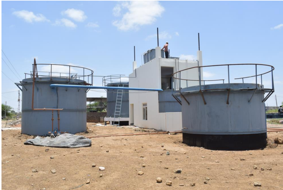
Fig.3: Secondary Clarifier & Settler-2
