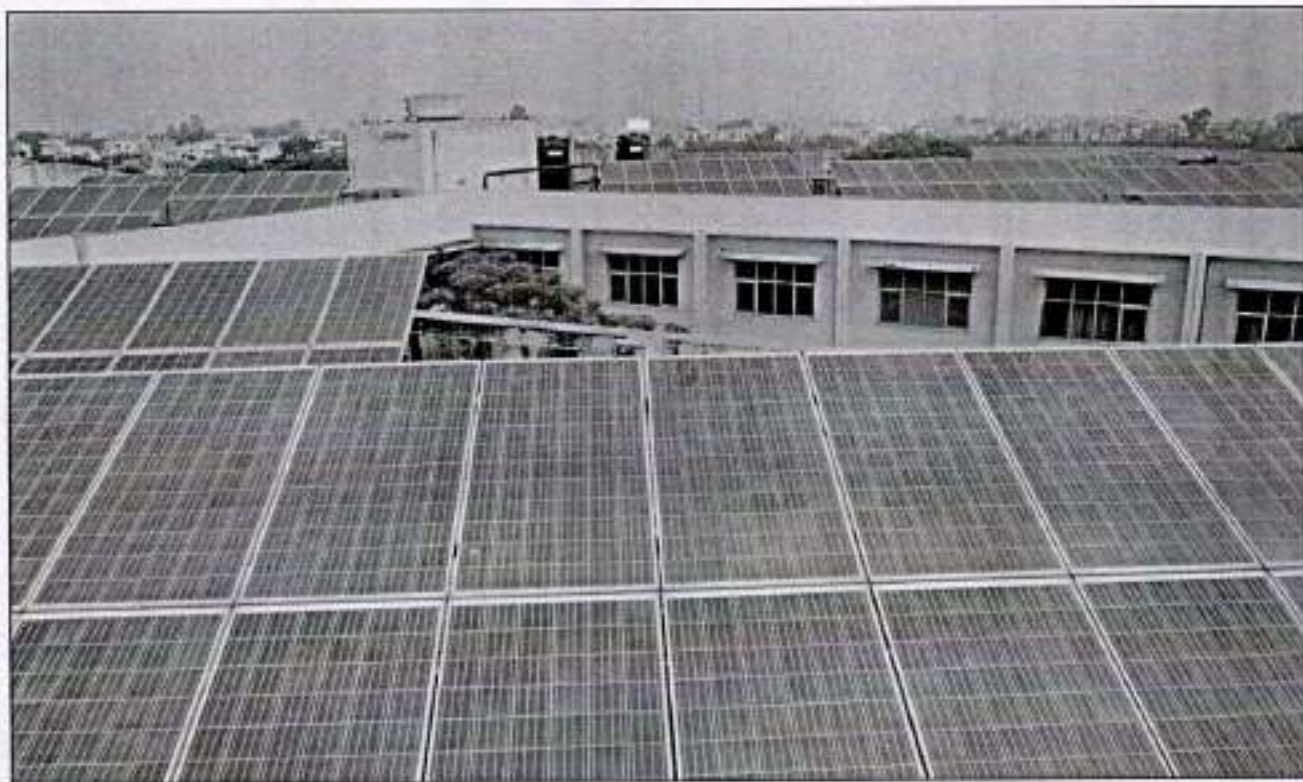
A view of the grid-connected Roof-top Solar Power Plant at NITRA in order to promote 'Green Power' in the industry
